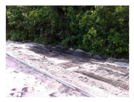
10. Sta 139+00 to 140+00 – Flooding across sidewalk into residential lots. EOR needs to check elevations at this location and provide revision to correct drainage problem:
