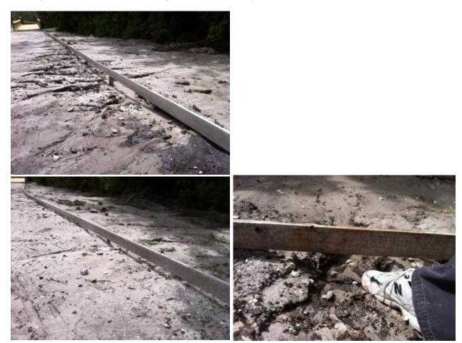
Cline's response to our request for them to remove the form boards, backfill to elevation, re-compact, and re-test for density, is listed below.
