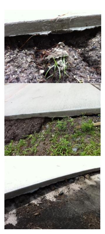
Cline's repair to date has been to backfill with loose soil and shove it in with their shovels and feet as observed on two occasions so far. The City has concerns that this does not meet specification and density requirements. Please advise the proper procedure for repair to achieve compaction density requirements in the case of undermining of the edges of the pathway. Click on the following link to show their repair technique from this
