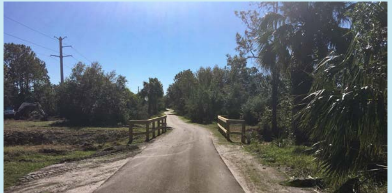
Public Works employees constructed the Forest Branch Path along the FPL easement from Old Kings Road to safely connect to Matanzas High School.
