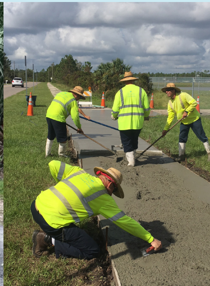
Public Works employees complete the resurfacing of the St. Joe's Walkway this year. Crews work hard to maintain more than 150 miles of sidewalks, walkways and bike paths.
