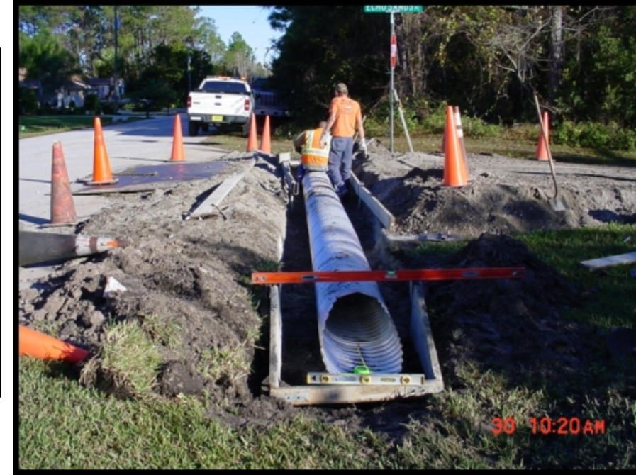
Valley Gutter Installation
