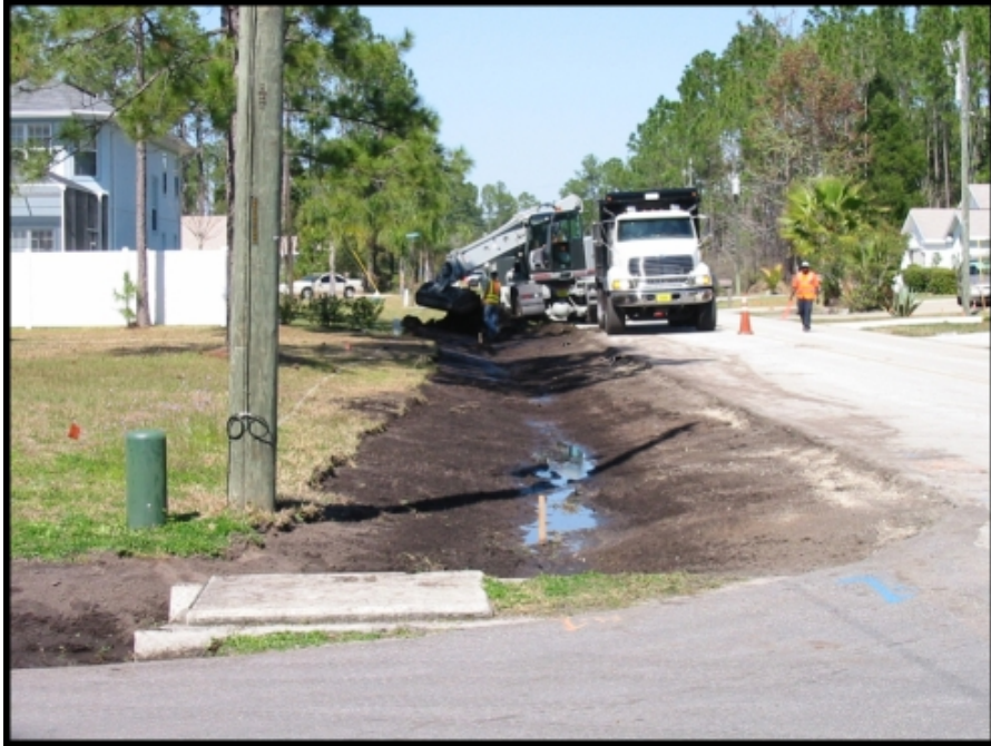
Swale Rehabilitation
