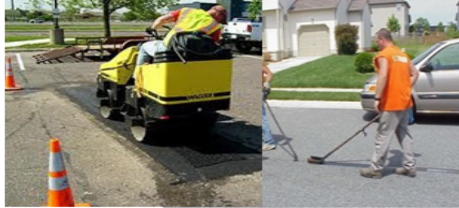
Patching/Crack Sealing
